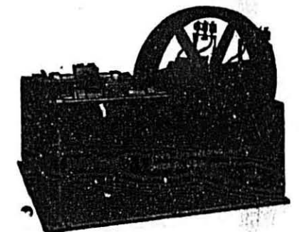
Four Plunger Horizontal Pump No. 9
